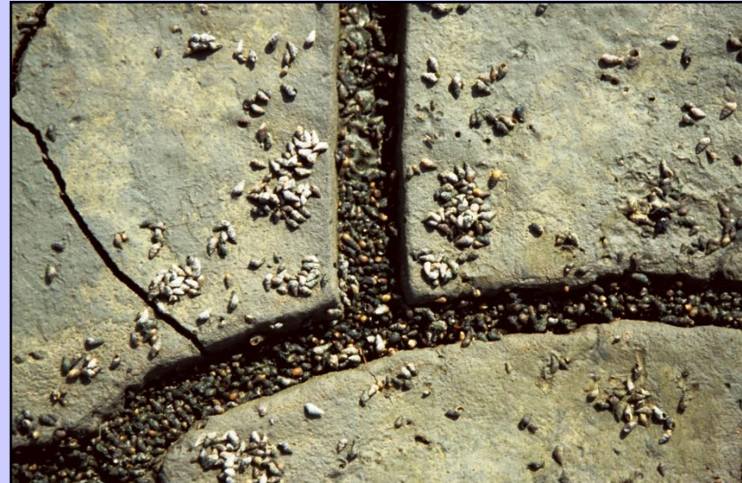
Cracks filled with tests of the snail Hydrobia
